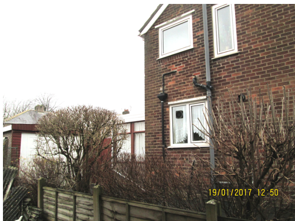
side of no.45 Prairie Crescent
