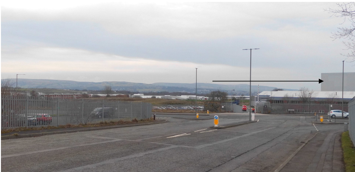
New building will be connect to the existing Phase 1 building
