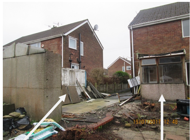
no.45 and rear of no.47 Prairie Crescent
