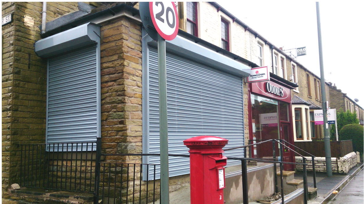
existing security shutters
